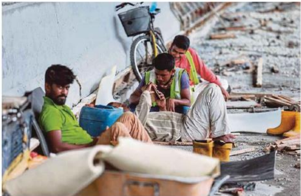
Migrant workers resting under a highway construction site in Ampang Jaya, near Kuala Lumpur, yesterday. PIC BY ASINAWI KILAS
