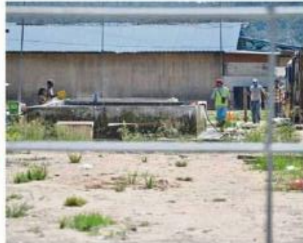
Foreign workers seen at a construction site in Puncak Alam.
