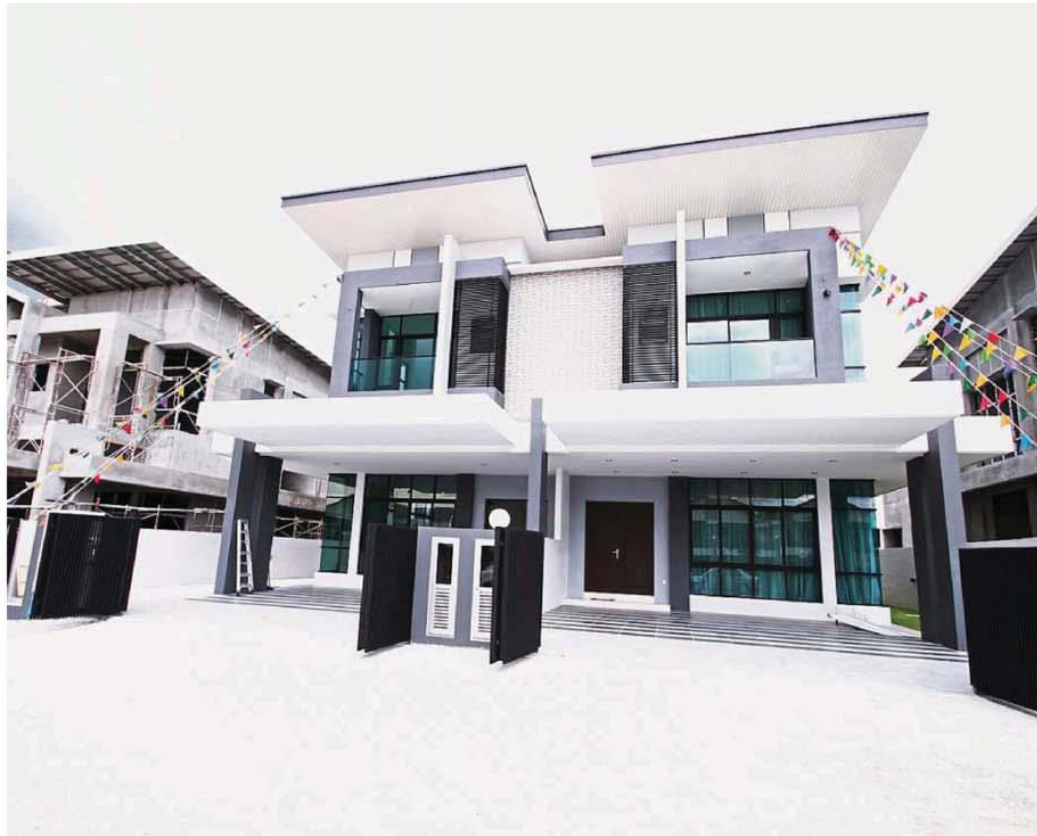
A show house of a new development in Ipoh.
