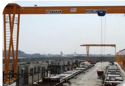
Production Yard at Setia Alam
