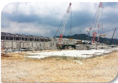
Precast Yard at Shah Alam North
