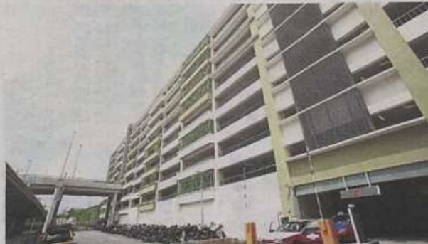
Worry free: The ample covered parking bays at the Sg Buloh station.
